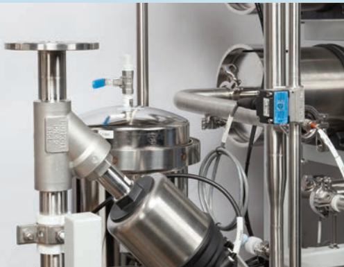
Automated self-adjusting modulating valves to control reject.
