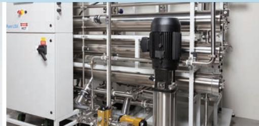
VFD Distribution Pumps reduce energy consumption.
