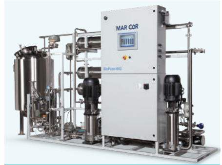
Modular skid system separates for easy installation.
