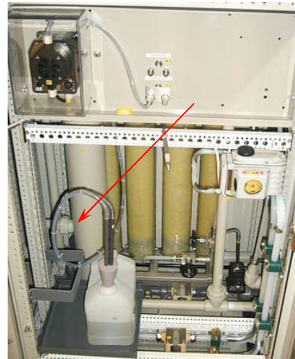
Inlet connection to low side port
