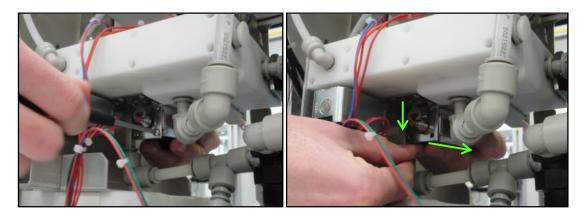
6. Remove the plunger from the solenoid and discard the existing spring.
