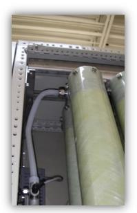
3. Remove the 4 nuts holding the top rails (angle brackets) in place. [The top rails support the upper manifold as it connects to the top of the housings]. Remove threaded rod nut on 104-106 machines.
