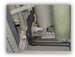
12. Remove manifold and lower support bars from the frame.
